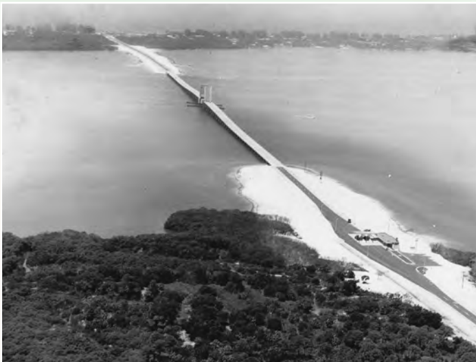
Manatee Bridge opened as a toll bridge in 1957. Toll collection ended in 1964. This photo looks from the mainland out to the Island. The toll booth can be seen at the bottom right. Kingfish Boat Ramp does not yet exist.
