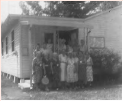
Harvey Memorial Community Church, April 1959. Generous church members and friends from the community have helped complete the many renovations through the years.
