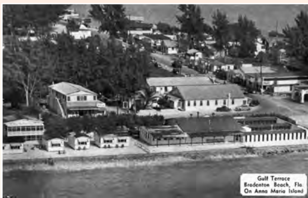
Gulf Terrace restaurant and Bradenton Beach bathhouse, ca. 1950. Photograph courtesy of the Manatee County Public Library System's Digital Collections.
